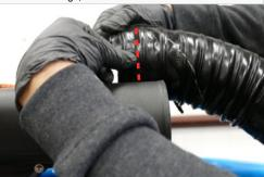
19. Pierce the Duct (P) centered between the two wire reinforcements using a razor blade to cut the duct to length. Cut all the way around. Try to cut the duct straight around the center as close as possible.
